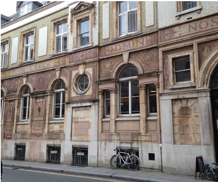
Figure 1: Sgraffito and terracotta detailing to building elevation Photo © Lighthouse Surveyors
