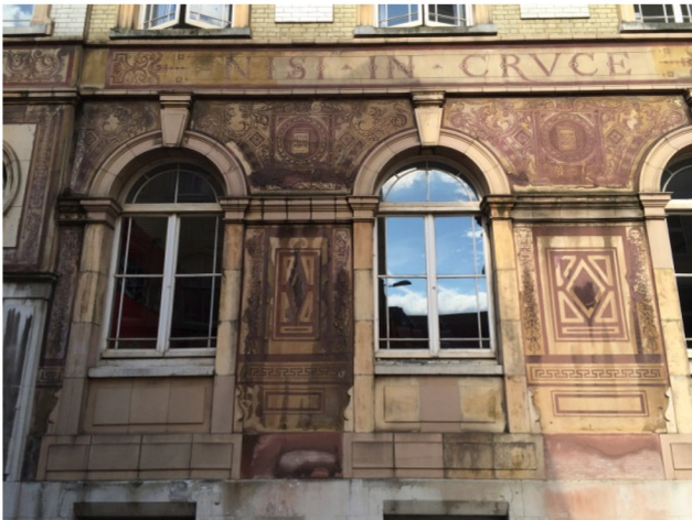
Figure 2: Severely weathered/perished sgraffito render Photos © Lighthouse Surveyors
