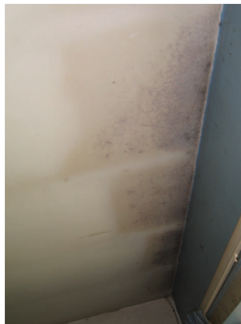
Figure 2: Above this ceiling, the loft insulation has not been pushed up to the back of the wall plate and taken over the head of the wall. Condensation and mould growth has formed on the resulting cold areas. This is still visible despite being cleaned with diluted bleach
