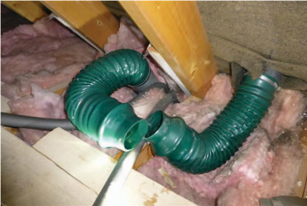
Figure 4: This flexible duct should connect the extract fan from the bathroom to the ventilating tile in the eaves of the roof. Because the wrong ducts have been used, it is impossible to join these effectively allowing warm moist air to get into the roof space
