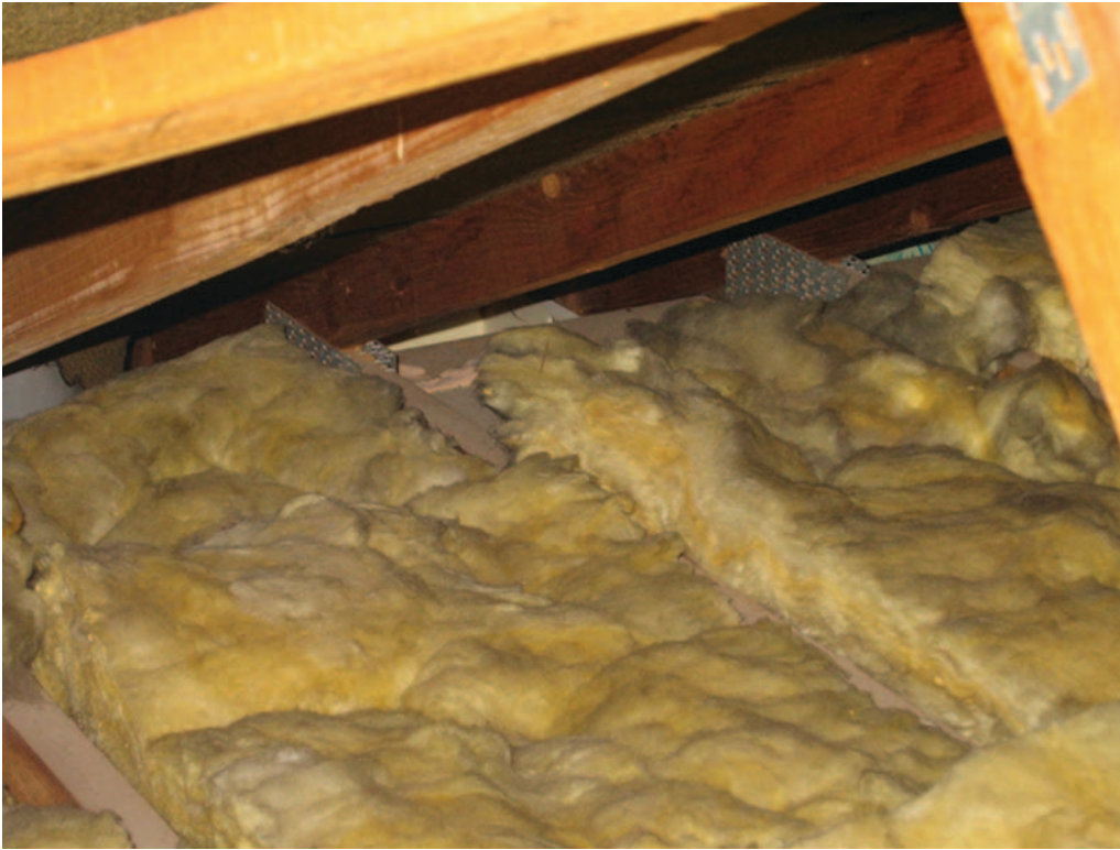
Figure 3: This is the view of the same ceiling shown in Figure 2 but from within the loft space. The insulation is approximately 75mm thick and upgrading this to 250–70mm while maintaining roof space ventilation would be a challenge
