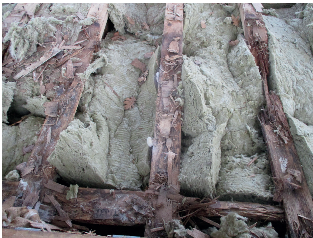
Figure 1: Example of extensive failure of roof deck to a private house — the effect of water entrapment in a cold roof
