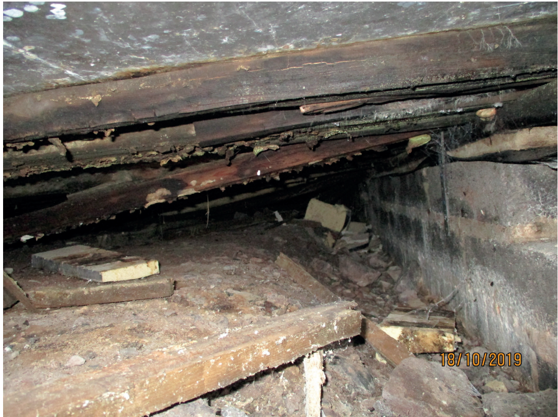
Figure 3: What happens when you do not ventilate a floor void properly
