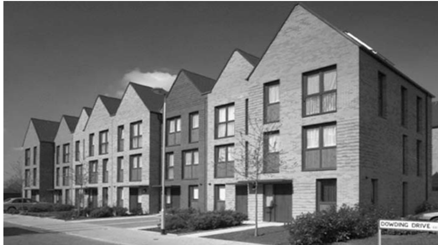
Figure 3: New family housing at Kidbrooke Village, London by Berkeley Homes
