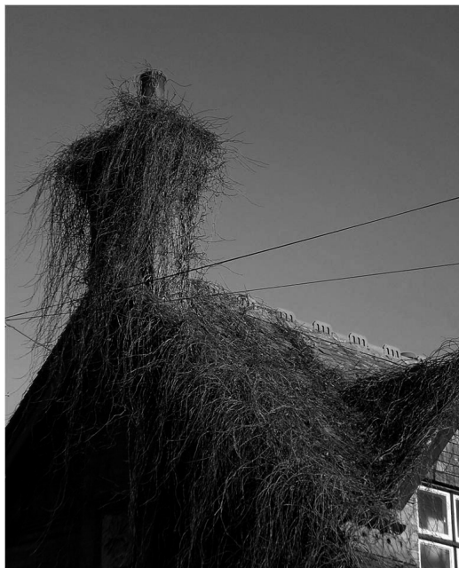
Figure 8: Example of long term neglect — a common cause of defects
