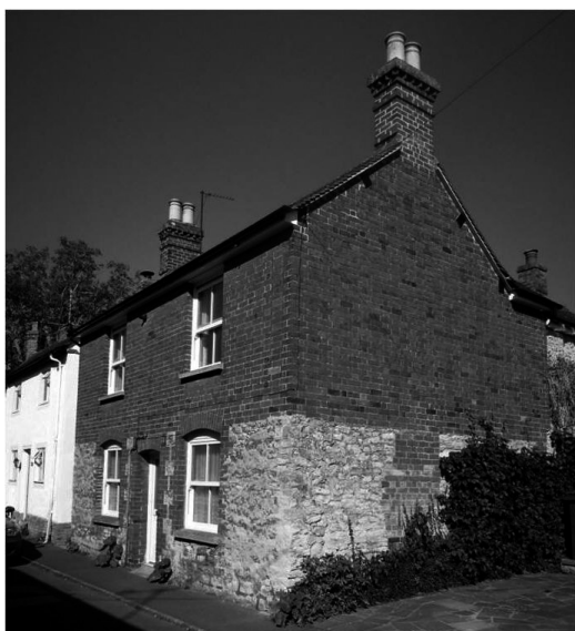
Figure 3: High ground levels are a common cause of low level damp
