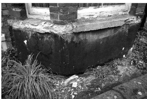
Figure 4: Extreme example of eroded sills resulting in damp to lower walls and floor structure
