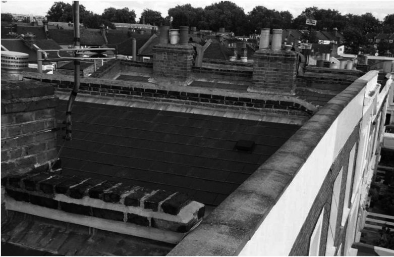
Figure 1: Parapet wall on a early Victorian 'butterfly' roof (aka 'London' roofs)
