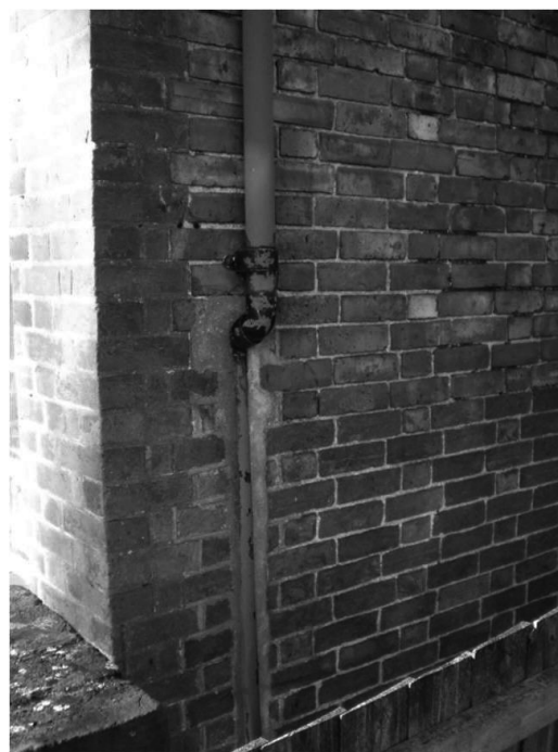
Figure 7: Embedded cast iron downpipe — an inherent defect dating from the time of construction
