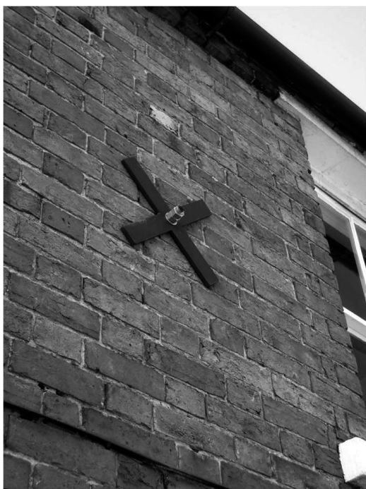
Figure 6: Traditional method restraint applied to bowing walls
