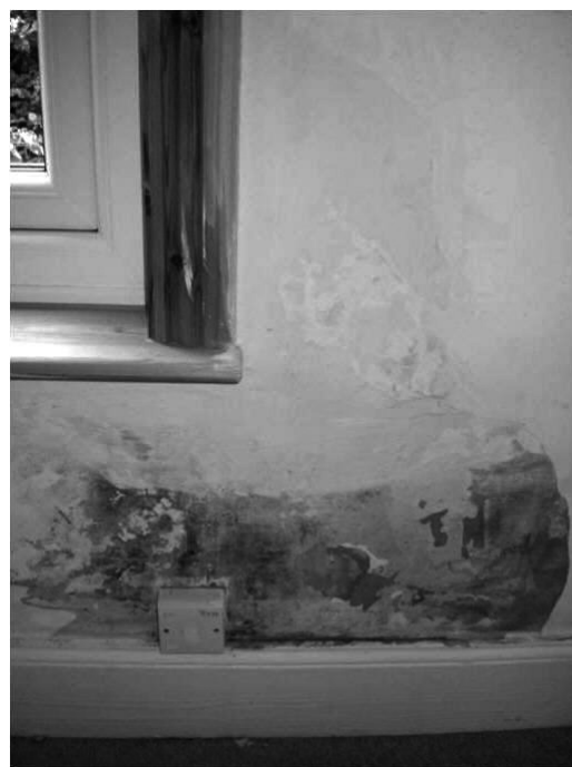
Figure 2: Damp — but not necessarily 'rising'
